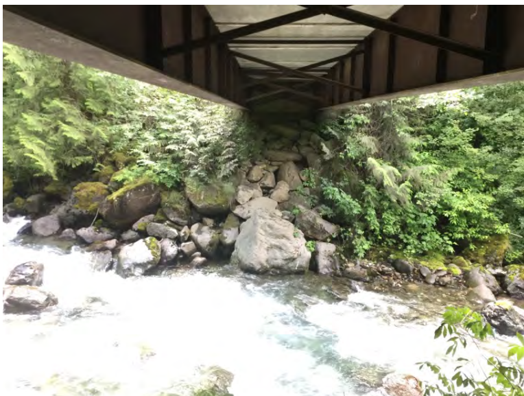
Left Bank Abutment when facing downstream
