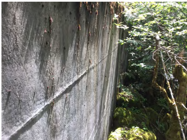
D/S right bank wingwall
