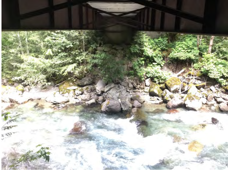
Right Bank Abutment when facing downstream
